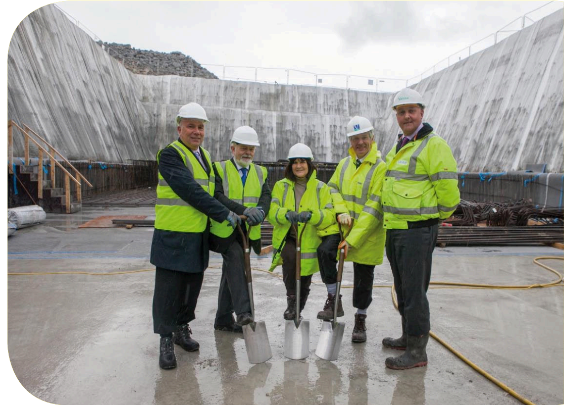
Start of construction of the Energy from Waste plant
